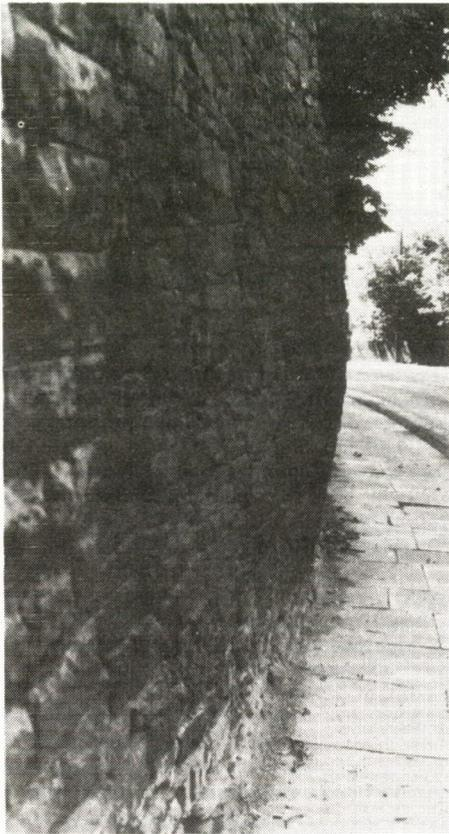
Fig. 6. Example of bulging on a rigid base — note decay of wall at base
