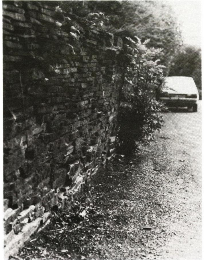
Fig. 11. Example of distributed sliding in wall retaining sloping ground
