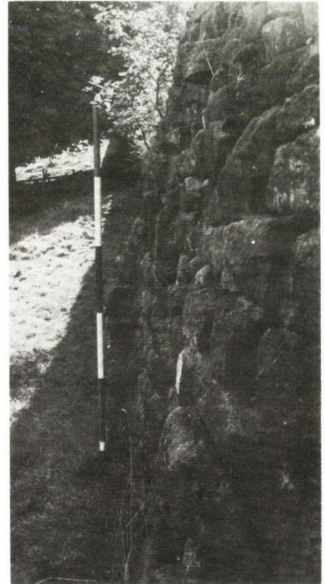
Fig. 9. Example of bulging due to inadequate bearing capacity
