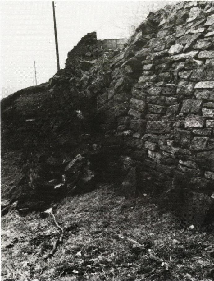
Fig. 10. Example of sliding on base, due to instability below wall
