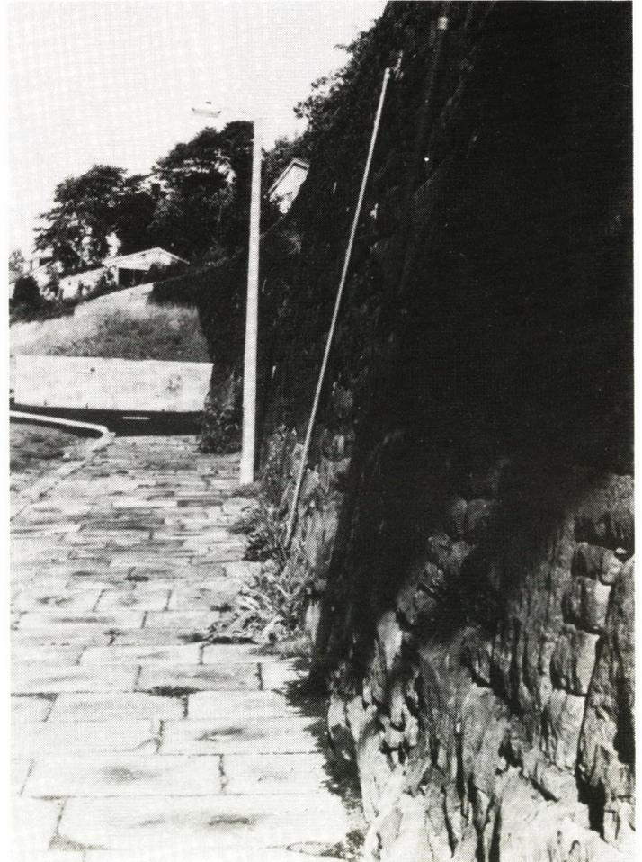
Fig. 2. View showing typical batter of dry-stone walls
