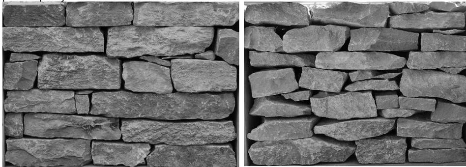
Figure 5: Sample wall blocks: a) best practice; b) poor construction
