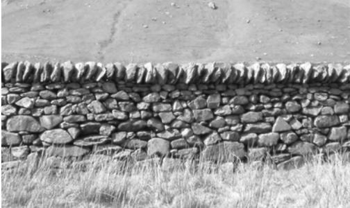
Above wall on slope showing jumpers and levelling.
